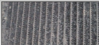
Evaporator before cleaning
